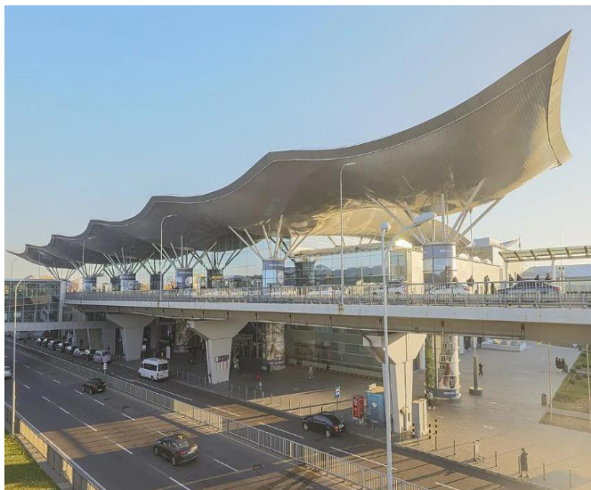
Figure 220. Boryspil Airport, modern appearance
