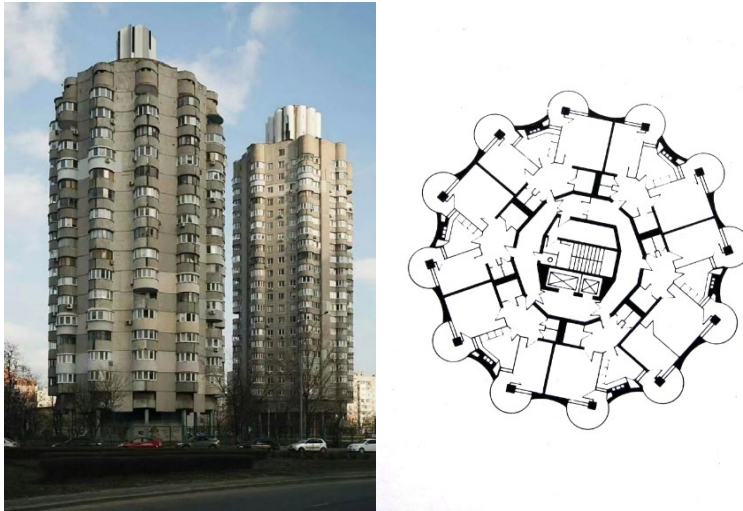
Figure 59. The Obolon Residential buildings
