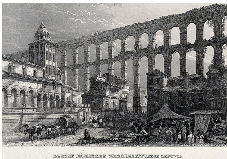
Figure 30. Roman aqueduct in Segovia, engraving
