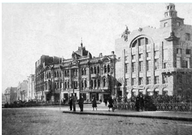
Figure 156. The Kharkiv Commodity Exchange, 1925 (architect V.A. Linetskyi)
