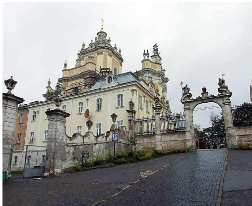
Figure 271. The complex of St. George's Cathedral
